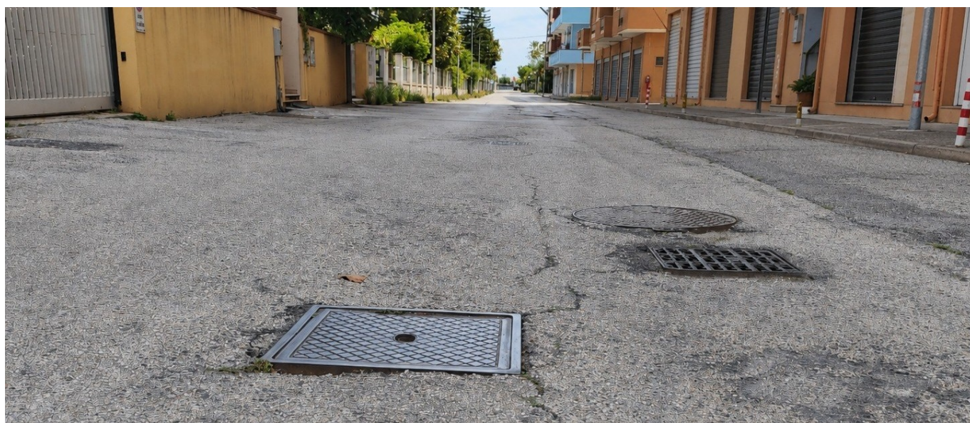
View of the urban area scanned: asphalt pavement, manholes and rainwater collection grate.
